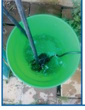
Also on March 3, 2022 the owner wanted to descale and flush his second tankless heater installed at his home, a Navien model MPE 210A. This Navien unit had been installed approximately 3 years ago and had also never been descaled and flushed. The chemical solution came out perfectly clear from the moment the chemicals started cycling through the tankless heater coils. No residual scale discoloration or debris of any kind was observed.
