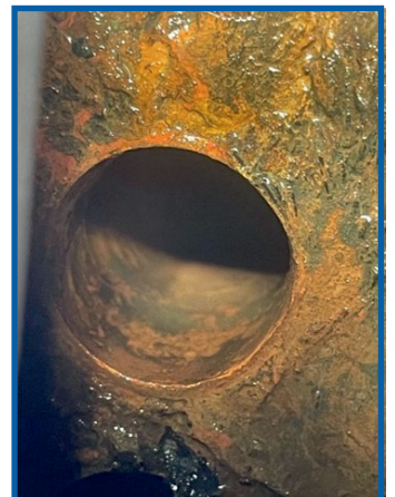
December 2021 - Condenser tubes remain scale free
