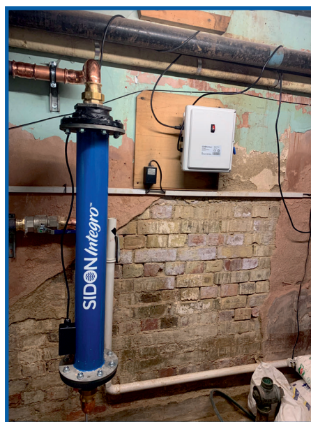
Integro™ 4 on the mains water supply
