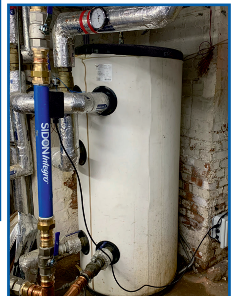
Integro™ 2 before the calorifier
